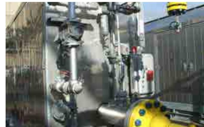
Given the parameters of incoming pressure, flow rate, inlet gas temperature of 35°F and the anticipated cooling from the pressure drop, the problem of solid hydrate formation was solved by technology developed by Bruest and proved in hundreds of installations worldwide. The technology is the Bruest HotCat catalytic infrared line heater.
