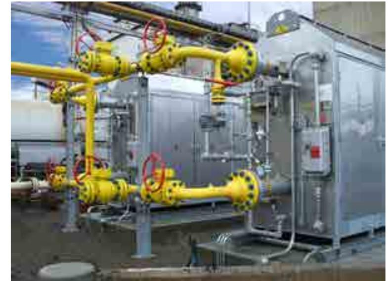
Two HotCat HC2000 catalytic infrared line heaters were engineered by Bruest, allowing the Pulp mill to replace costly oil with natural gas.
