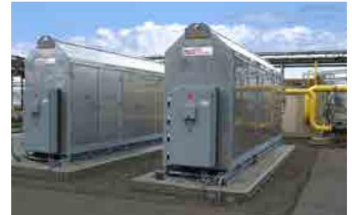
Two HotCat HC2000 line heaters were installed to operate in parallel. Though either unit could accommodate the mill’s nominal daily load, the mill purchased two units for redundancy. It is fortunate they did, for on a tough day in late 2012 the mill had to run both units “full-out” to keep the mill’s boilers fed with natural gas.
